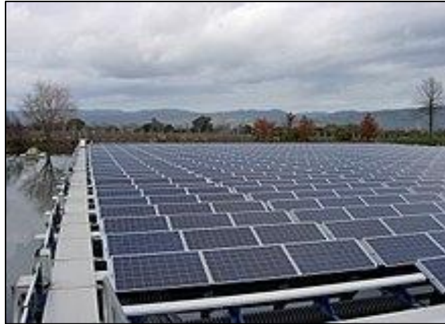
Fig. 13. Floating photovoltaic on an irrigation pond [58]
