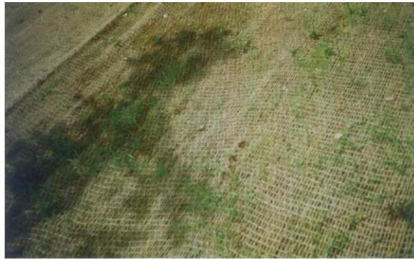
Fig. 3. Coir netting used in soil stabilization [8]
