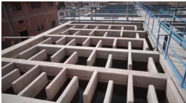
Fig. 6. Hydraulic flocculation chamber [5]
