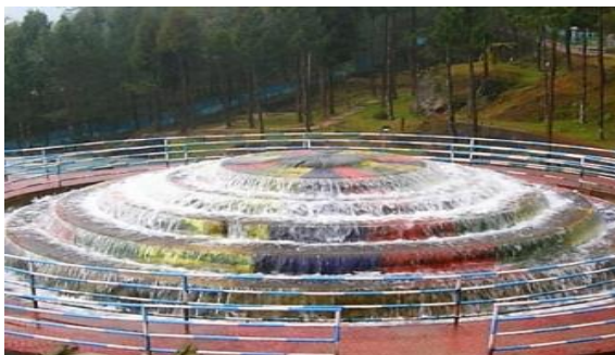
Fig. 4. Cascade aeration type 1 [4]
