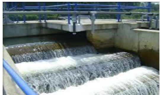
Fig. 5. Cascade aeration type 2 [4]
