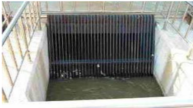
Fig. 2. Coarse screen [3]
