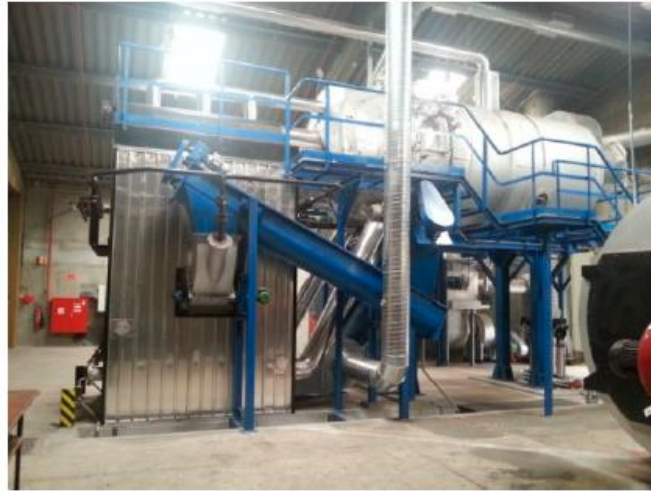
Fig. 32. The biomass steam boiler of a textile production plant [67]
